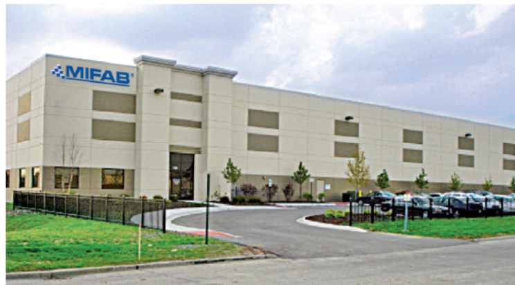
MIFAB's factory in Chicago, Illinois
